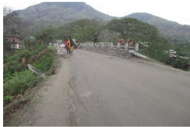
RoB at Chainage 6+641
