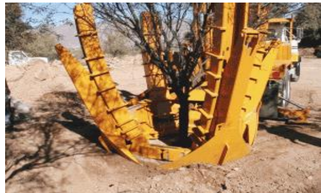
The blades are hydraulically inserted into the ground one at a time
