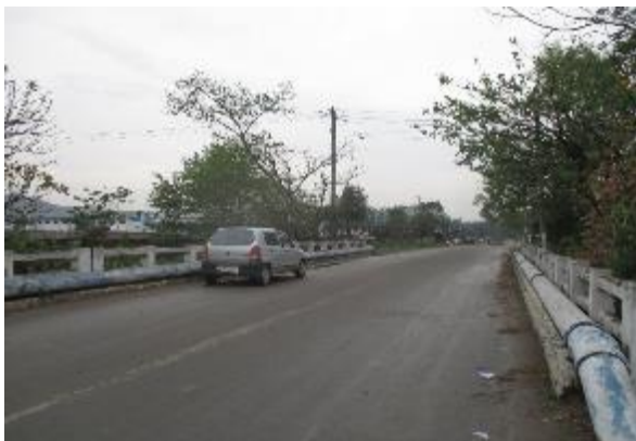
Minor Bridge at chainage 5+498
