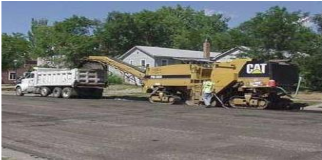
Figure 4.1: Milling of existing asphalt pavement
