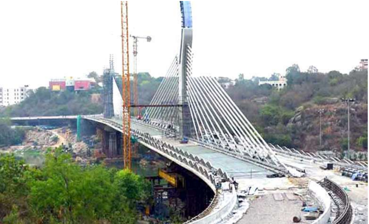
Fig: 4.6 Durgam Cheruvu Extradosed Bridge -Construction Stage
