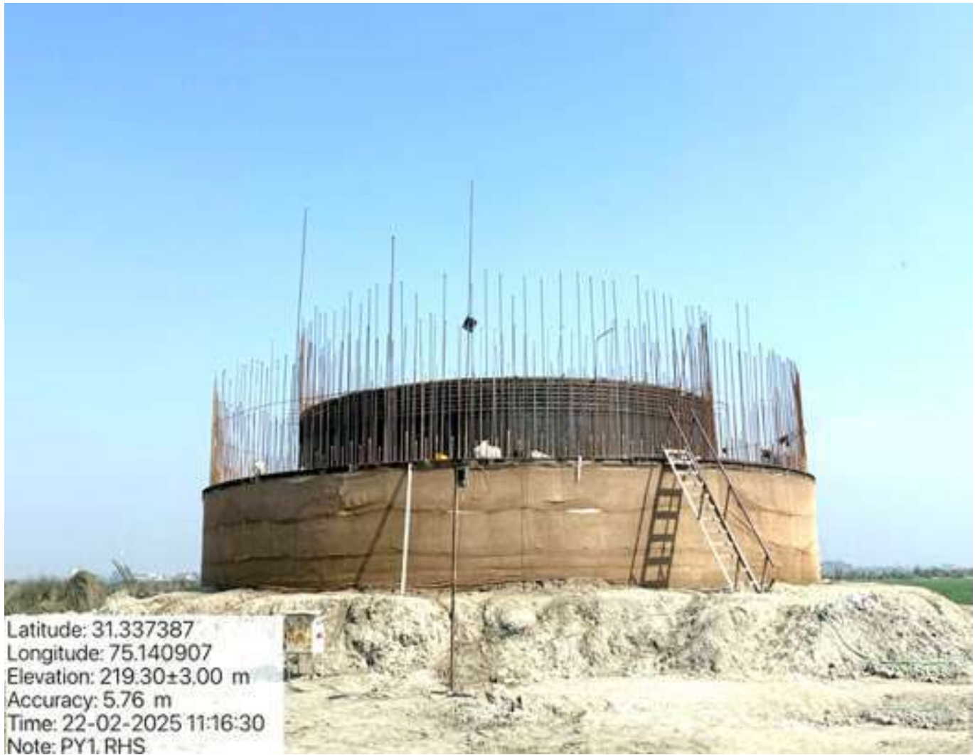
Figure15: View of Under construction main pylon well foundation.
