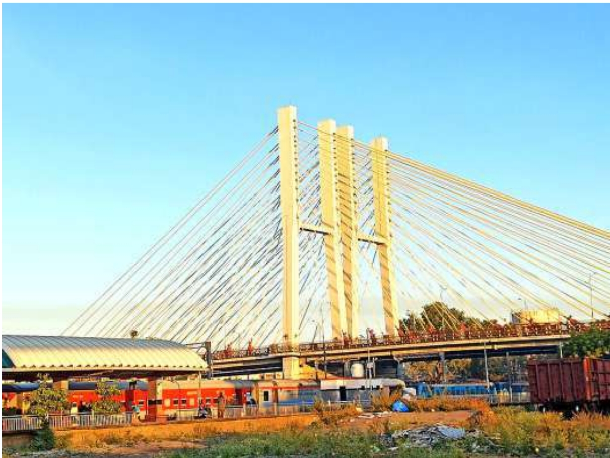
Fig: 4.2 Nagpur Cable Stayed Bridge
