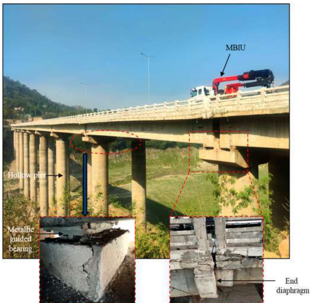
Figure 2. Detailed inspection of the remote locations of Major bridge @ Km. 26+100 (Kiratpur- Nerchowk project) using MBIU
