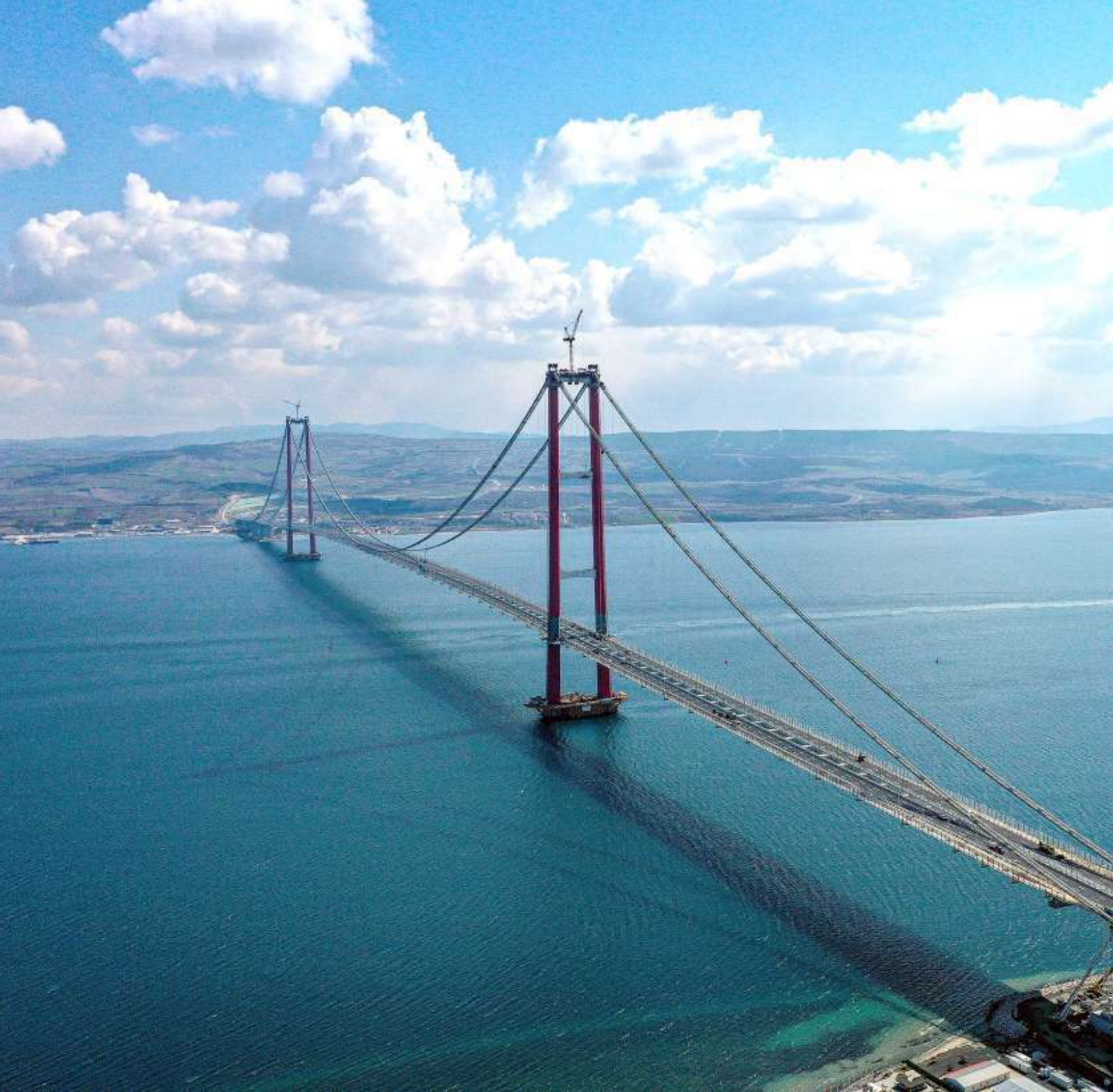
Figure 6: 1915 Çanakkale Bridge, Longest Suspension Bridge in the world (2033 m Main Span)
