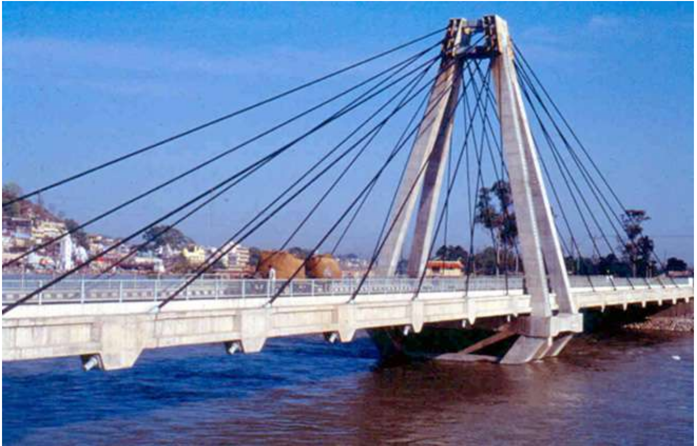
Figure 11: Haridwar Bridge - First in India
