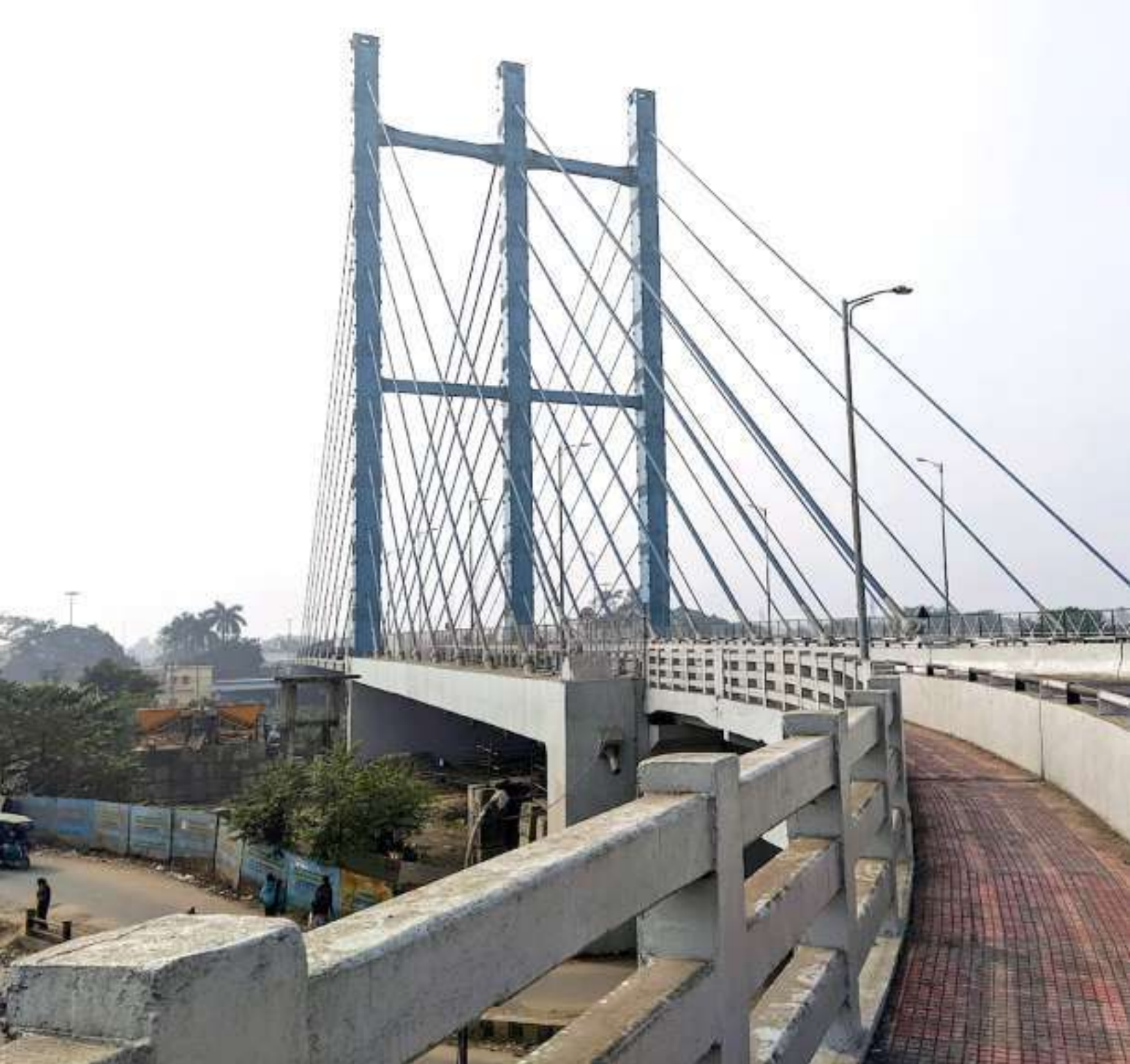
Fig: 4.5 Bardhaman Cable Stay Bridge
