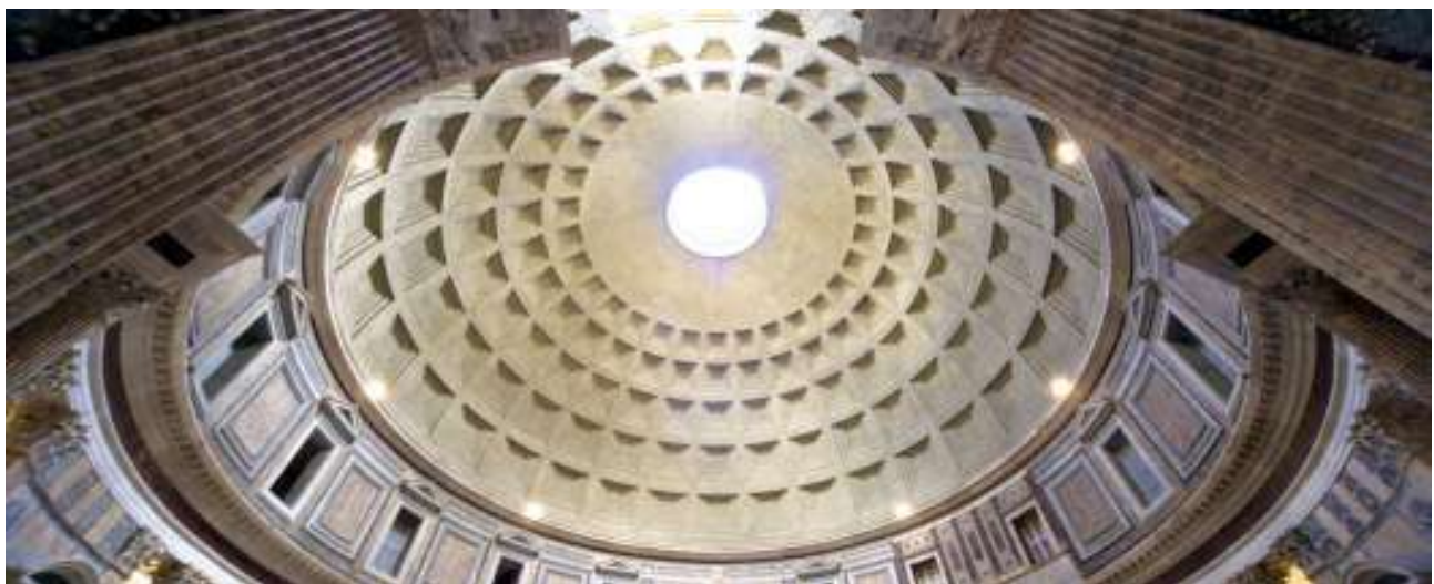
Figure3: The Pantheon at Rome using 'Hot mixed' pozzolanic concrete, with incredibly high strength
