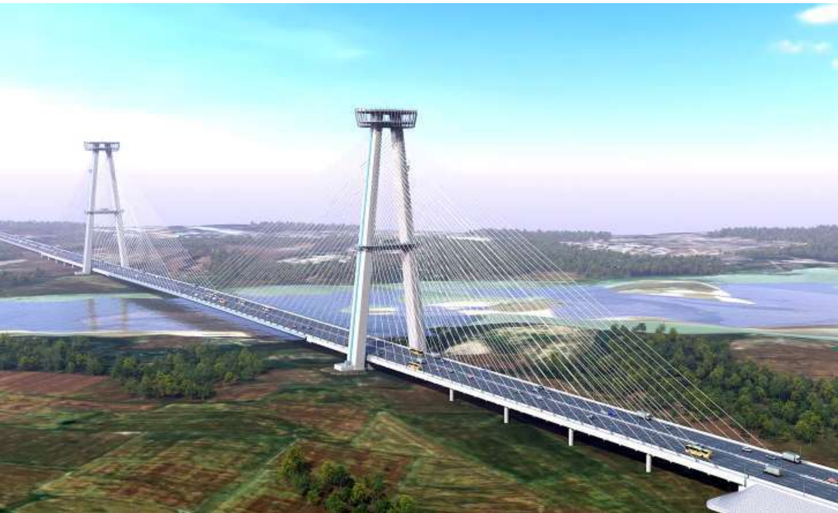
Figure14: An overall view of the Kapurthala bridge.
