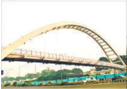
FIG 1. Steel Arch FOB of 90m span. concept comprises a steel arch bridge. No support at the central verge, provides enhanced safety from errant vehicles.
