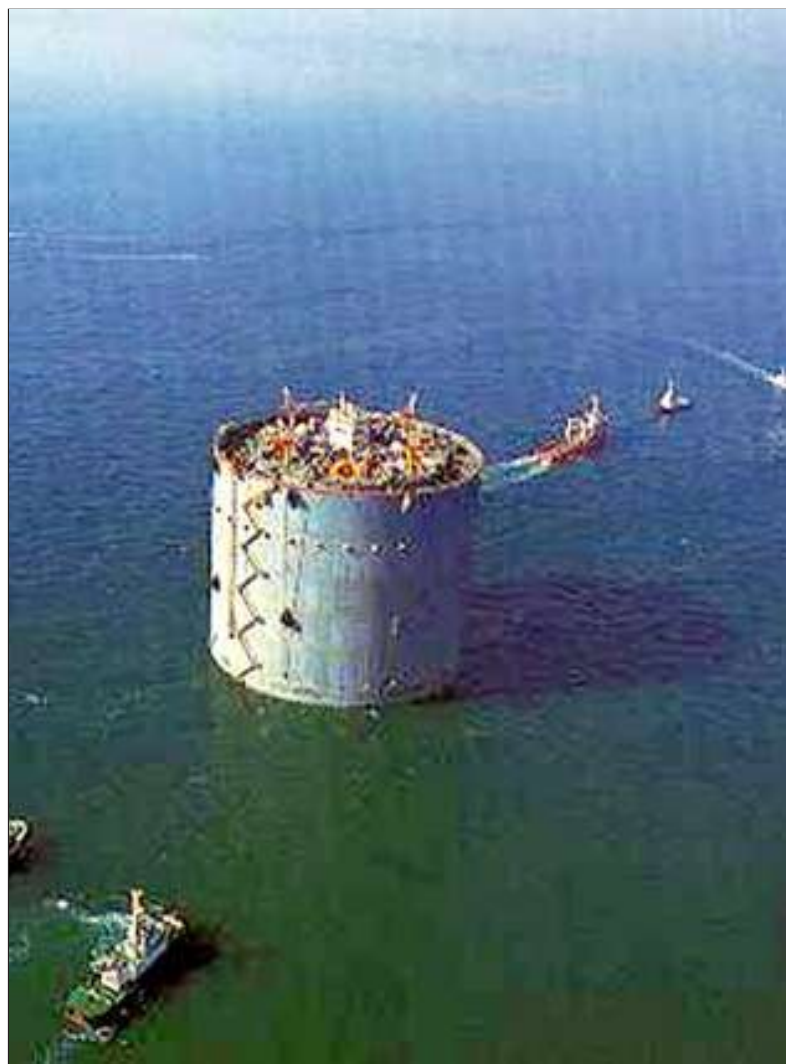
Figure 8: 80 m diameter steel caisson fabricated onshore being floated to the location of the pylon for the Akashi Kaikyo bridge
