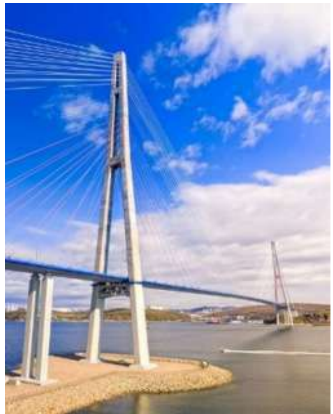
Figure 5: Russky Bridge, Longest Cable Stayed Bridge in the world (1104 m central span)
