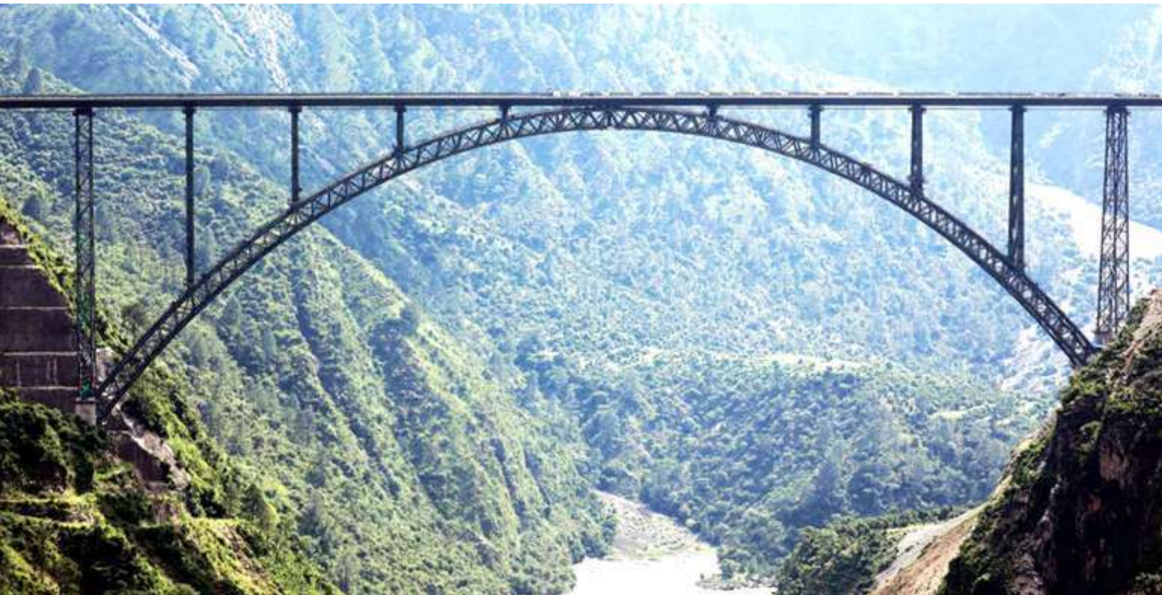
Figure 10: Chenab Railway Bridge - The highest in the world, Above bed level at 359 m
