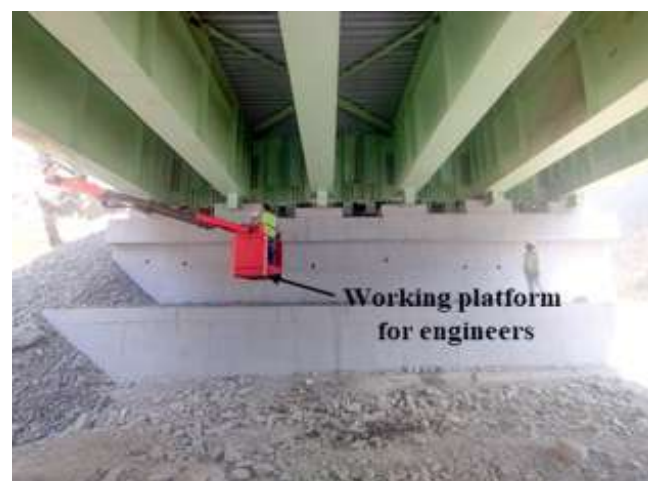
Figure 1. Physical inspection by bridge division staff of M/s ICT Pvt. Ltd. using MBIU (Z-morh)
