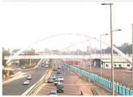
FIG 1. Steel Arch FOB of 90m span. concept comprises a steel arch bridge. No support at the central verge, provides enhanced safety from errant vehicles.
