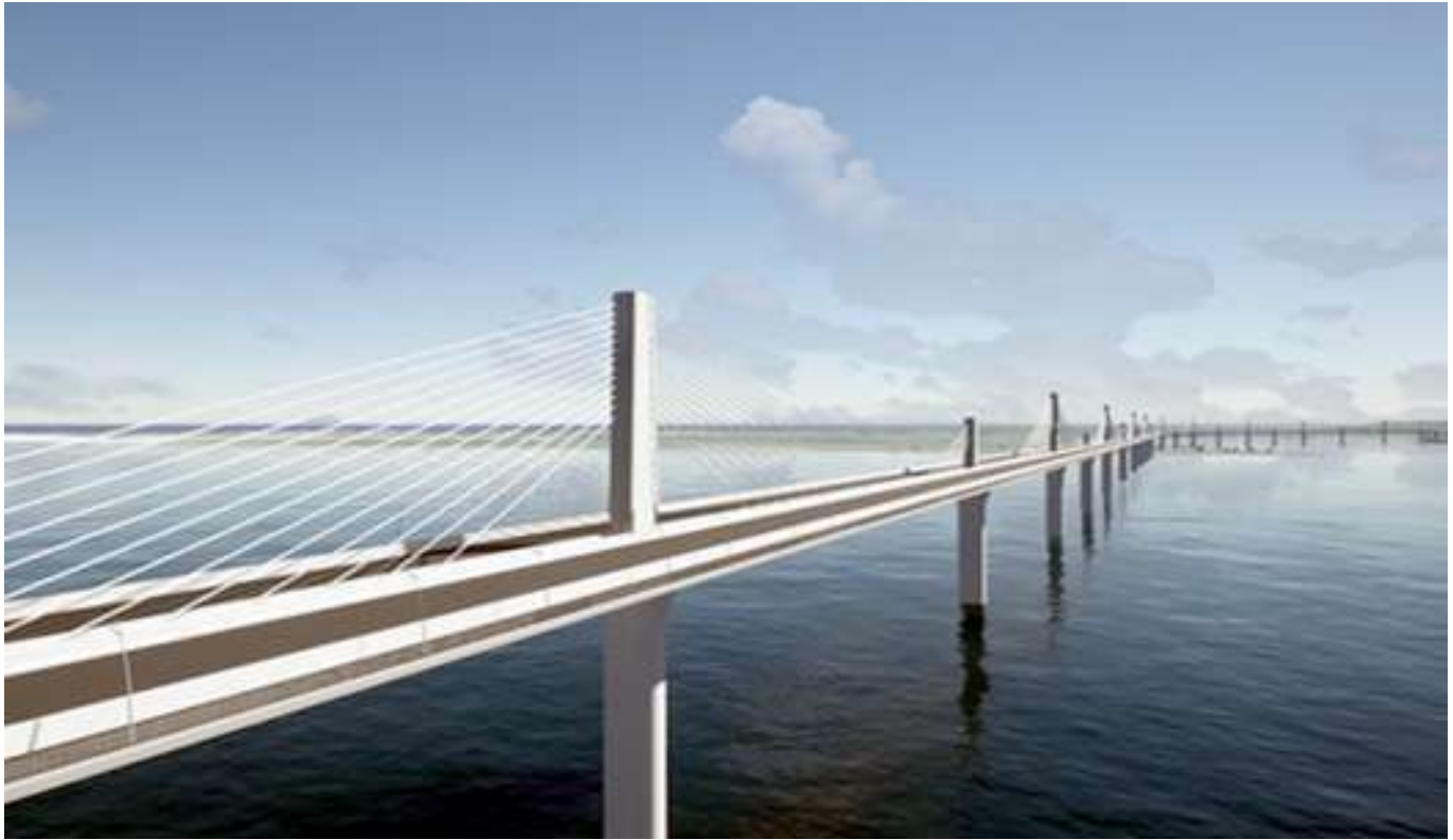
Figure 16: An overall view of the Palasbari bridge.
