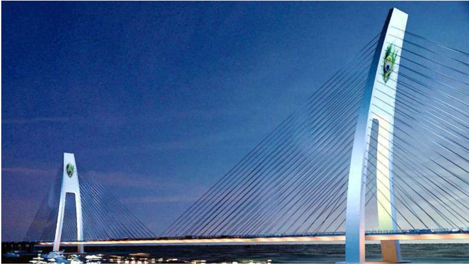
Figure 13: Okha-Bet Dwarka Signature Bridge-Longest Main span in India (500m) Completed 2024.
