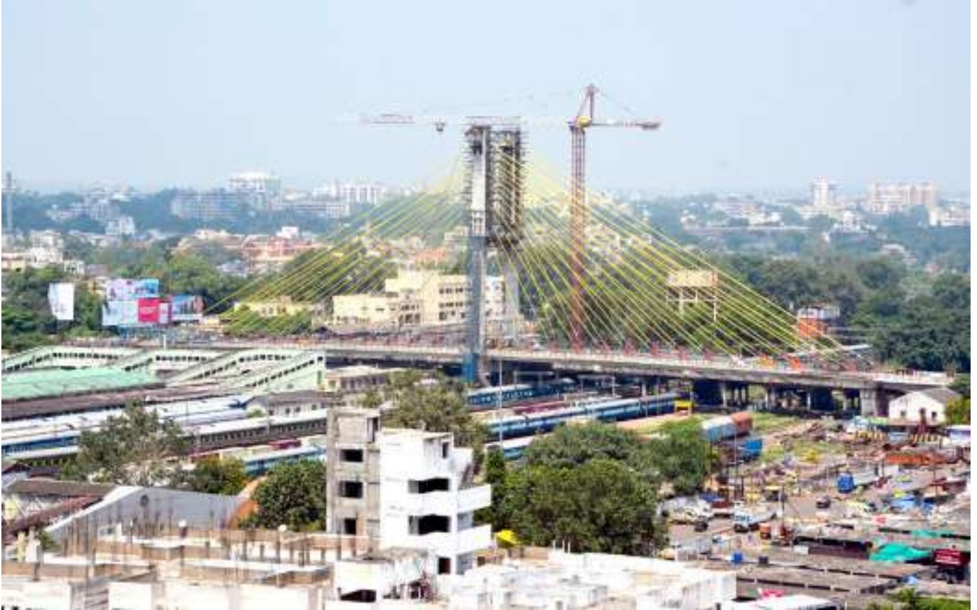
Fig: 4.1 Nagpur Cable Stayed Bridge -Construction Stage
