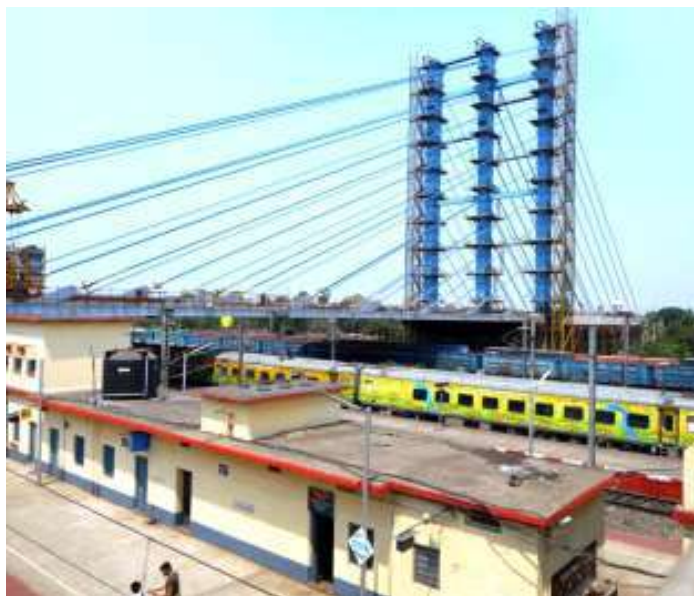
Fig: 4.4 Bardhaman Cable Stay Bridge - Construction Stage
