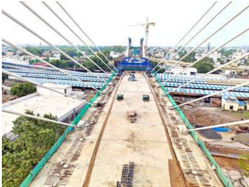
Fig: 3.2 Jabalpur Extradosed Bridge- Construction stage.
