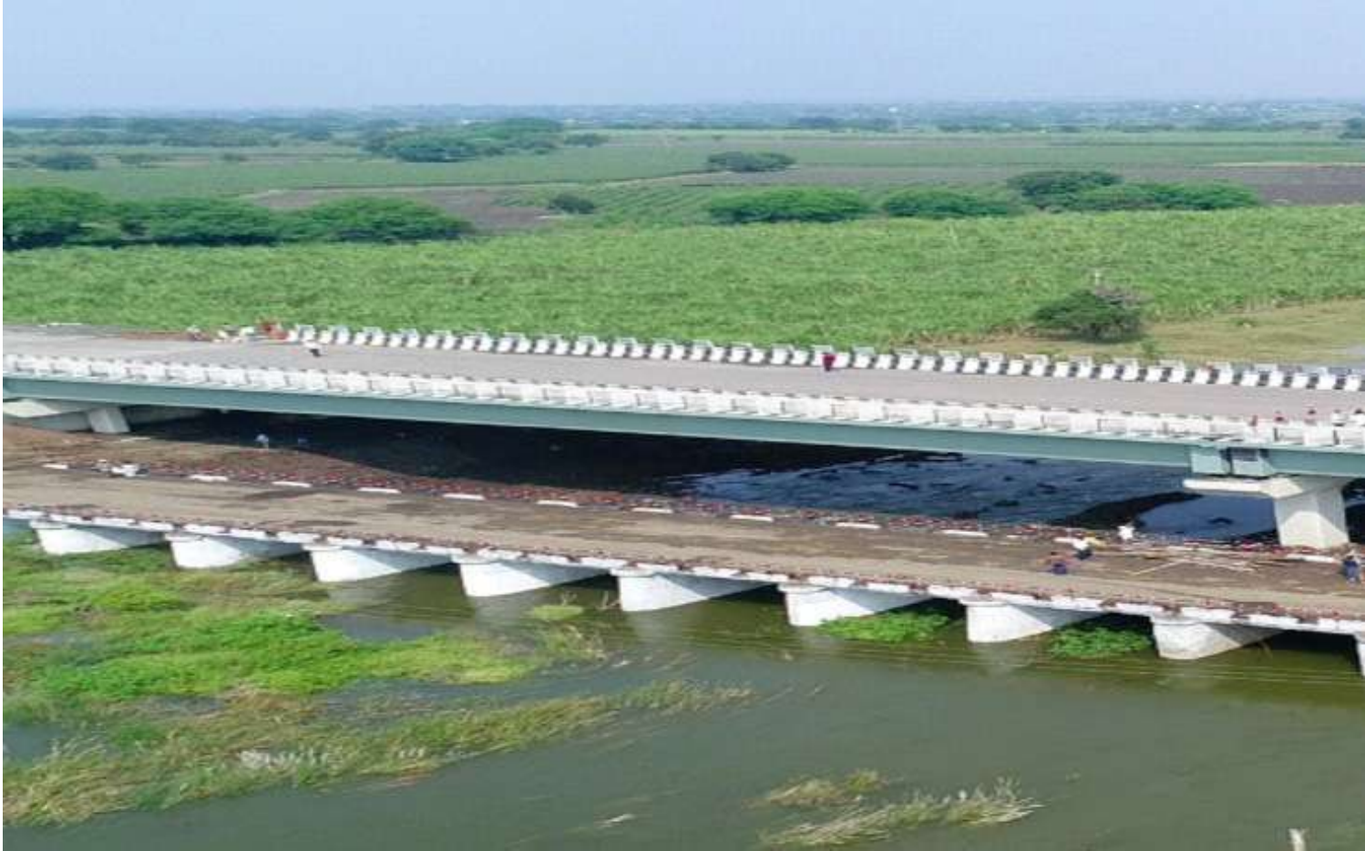
India's First Major Bridge Construction using UHPFRC Technology at Km. 42+050 on Sole River, Latur Nilanga Aurad Section of NH-752K, Maharashtra. Executed UHPFRC Long span configuration (02 x 56m). Source: Long Span Structures Pvt. Ltd., India.
